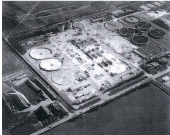
Figure 1.8 – Overview of a WWTP (under construction)
