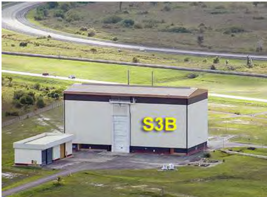
Figure 6.2.2.2.b – S3 area overview
