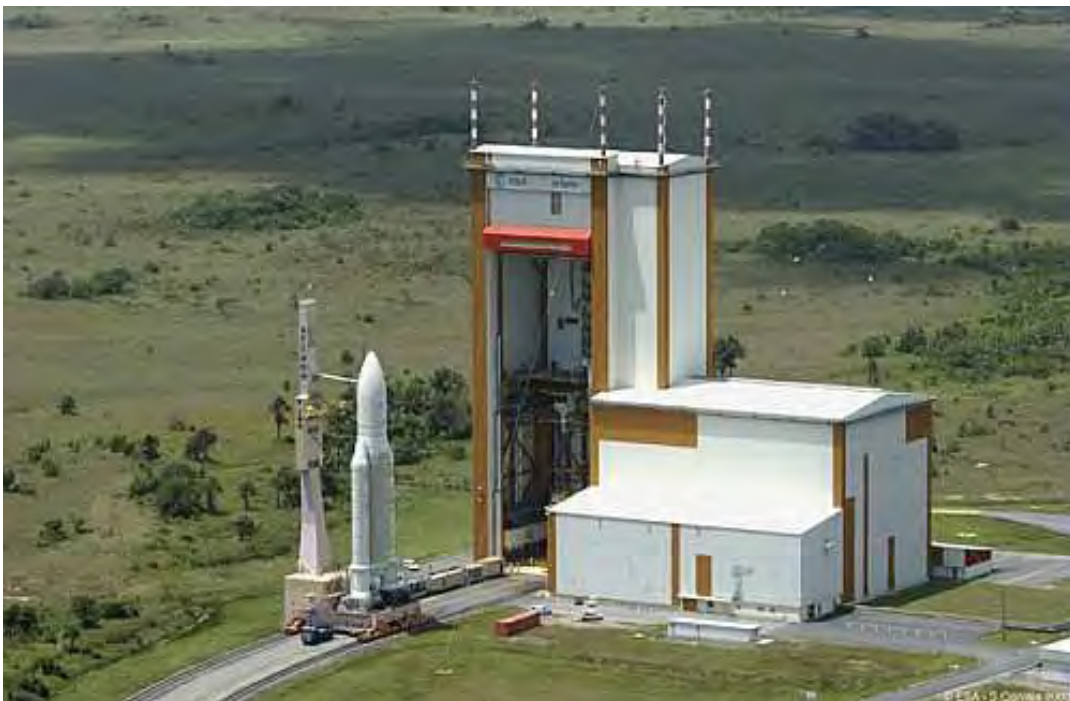
Figure 6.2.3.1.1.a – BAF launch vehicle access side
