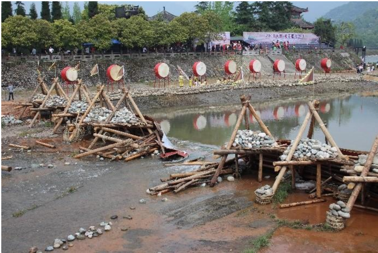
The main inlet has been opened. The irrigation season can start.
